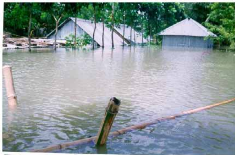
Bamboo protection wall to protect the from the movements of engine boats. Photo collected by Zonal manager, Faridpur
