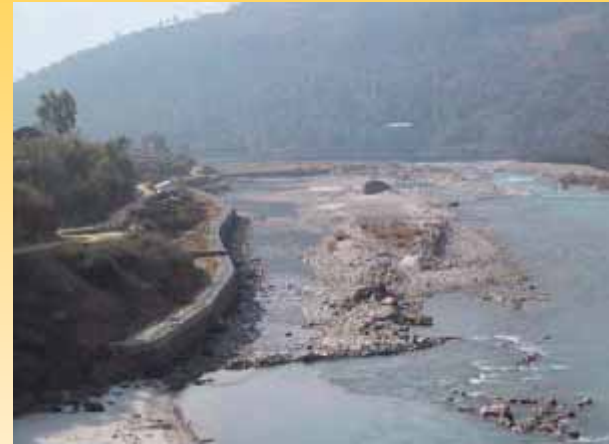
Protection against GLOF in northern Bhutan
